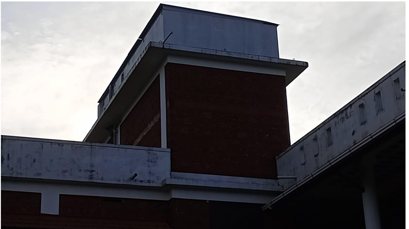
The Cement Concrete Water Tank over the New Academic Block
